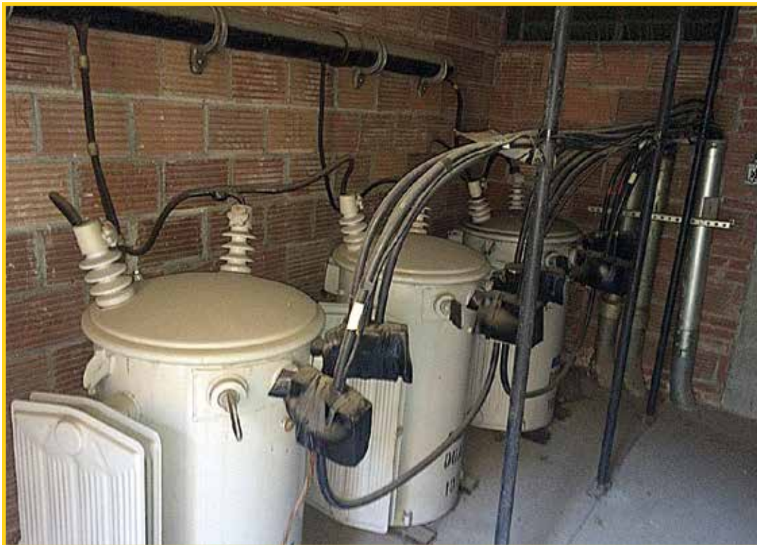
Electric service upgrades - The proposal includes plans to replace/abate old asbestos wiring at both the Jr./Sr. and elementary buildings along with miscellaneous other work.
